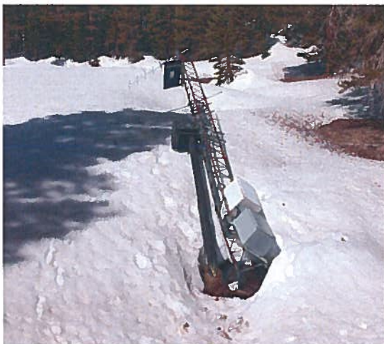
Photograph 1: Broken tower in Wet Meadow.
