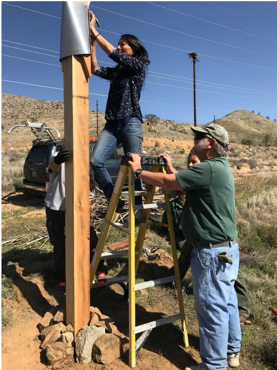
Figure 7. Tania Ellersick, Deputy District Ranger for Kern River Ranger District, staples predator excluding flashing to the nest pole.
