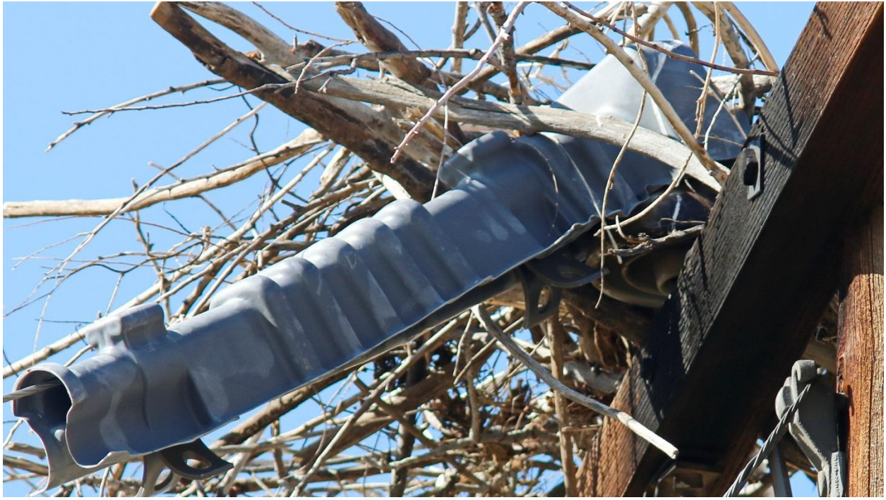
Figure 1. Burned pole with nest excluder.
