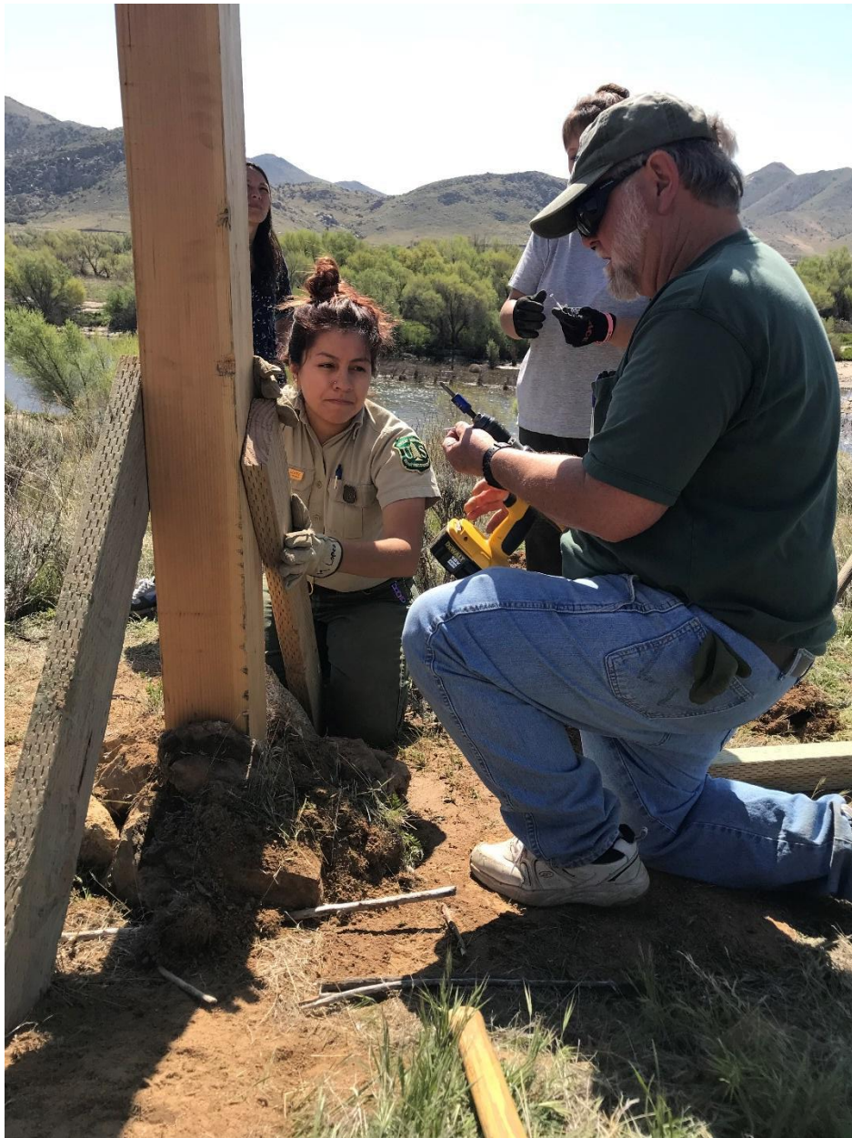
Figure 9. John Good adds supports to stabilize the new pole with assistance from Marcella Lopez.
