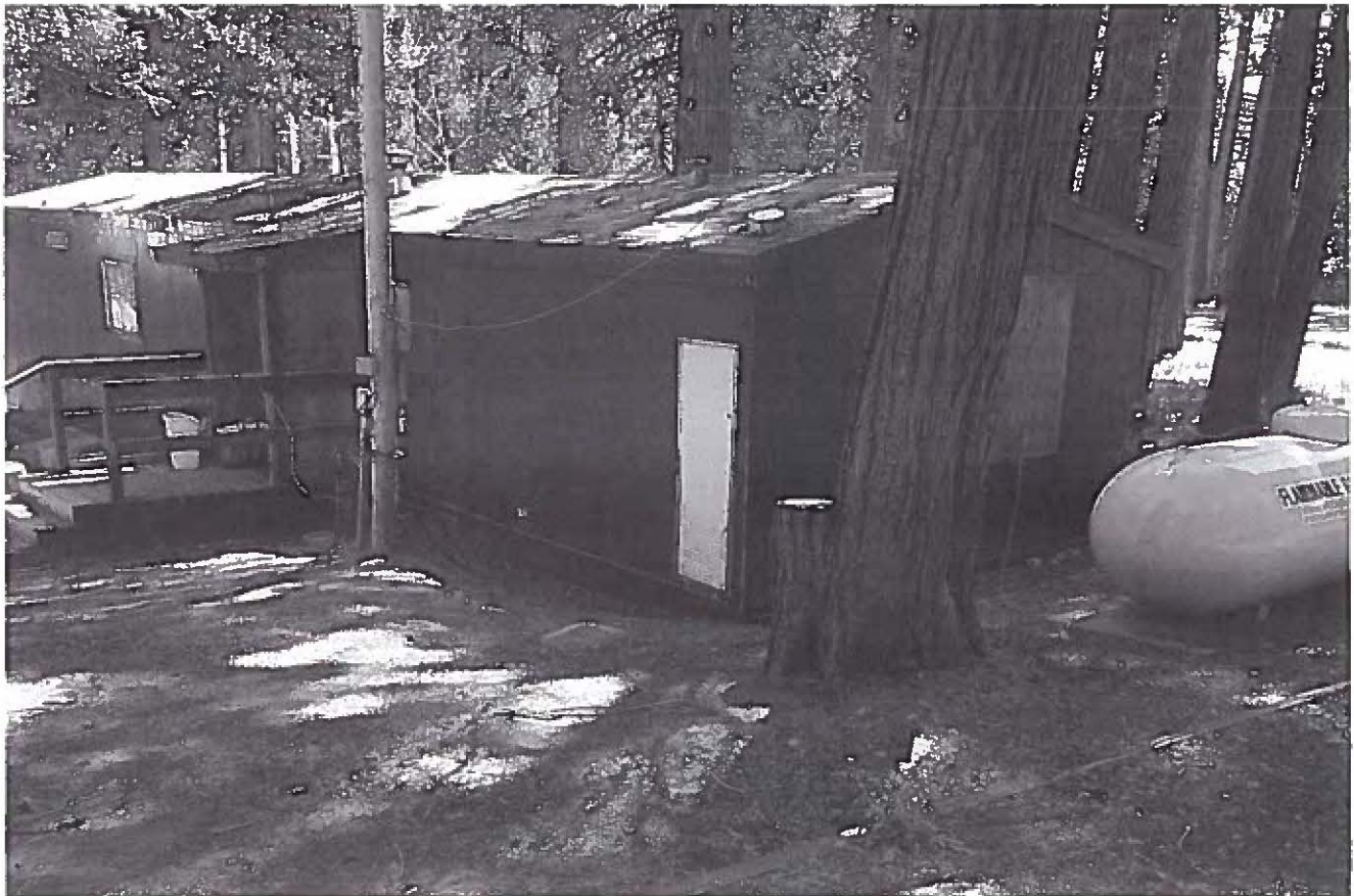
Fire Barracks Building (1231) proposed for demolition
